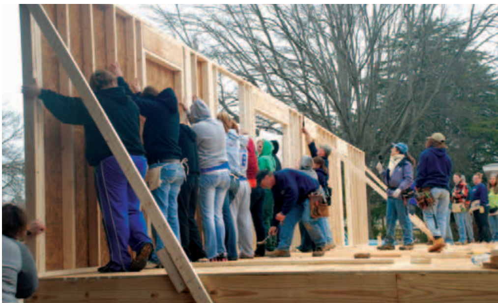
SWU's softball team helps build a Habitat for Humanity house in Liberty, S.C.
